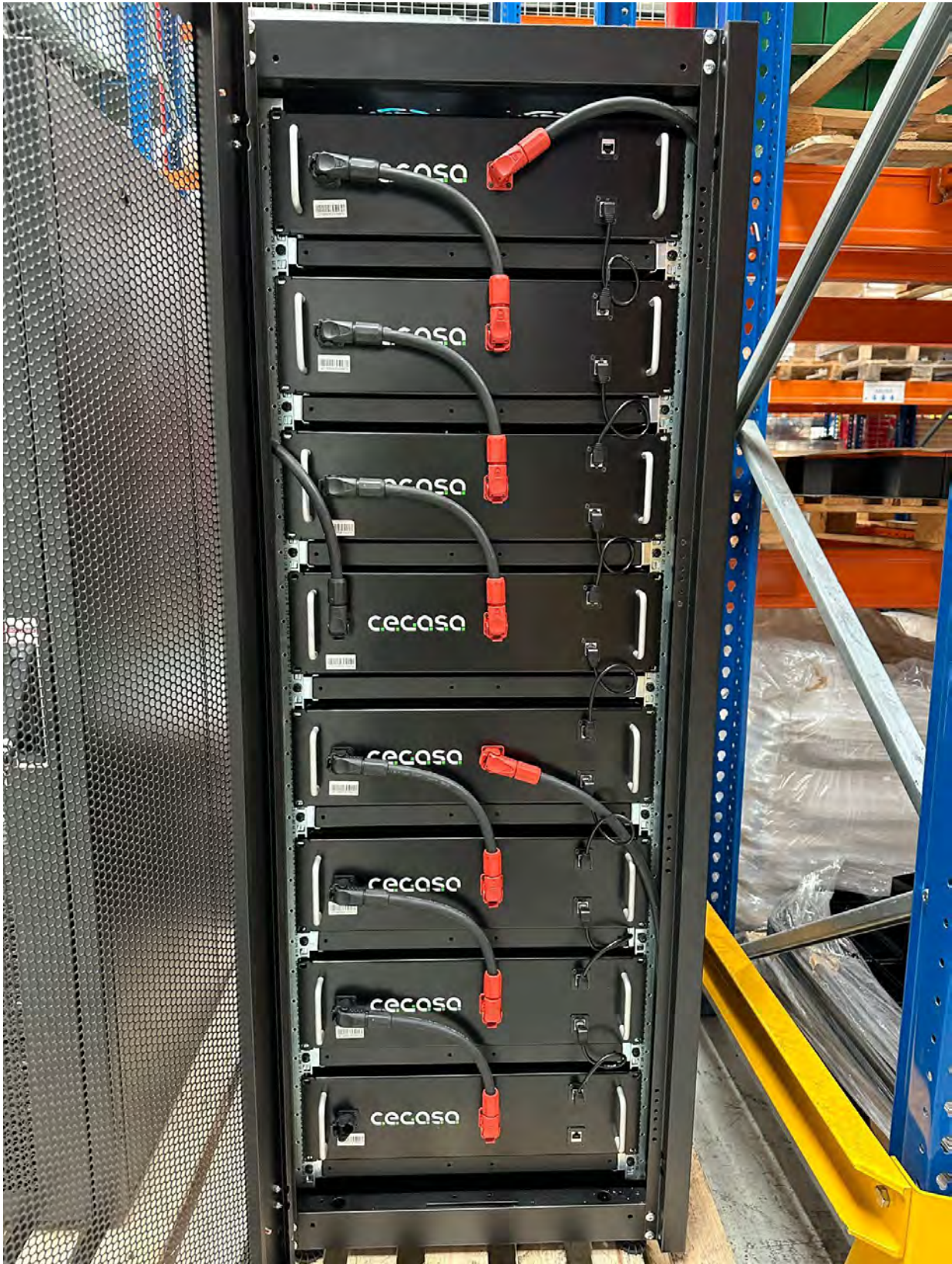
Figure 15. High-power battery string
